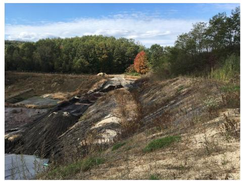
Photo 2: Landfill working face with benched slope constructed. The photograph was taken from near the top of the active cell and looking west.
