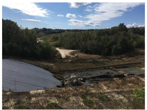
Photo 4: Landfill area not currently being filled (grassy area between leachate collection building and concrete barriers). The liner is visible on the left side of the photograph. The photograph was taken from near the top of the active cell and looking southwest.
