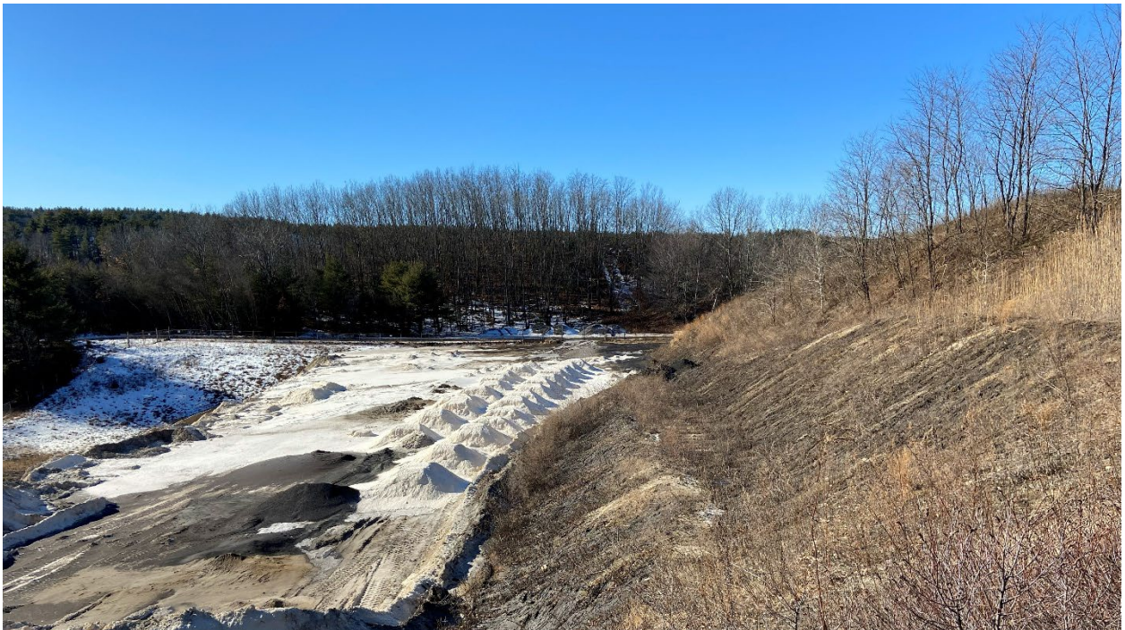
Photo 2: Landfill working face with benched slope constructed. The photograph was taken from near the top of the active cell and looking west.
