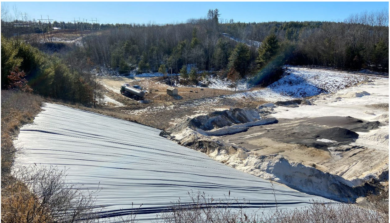
Photo 4: Landfill area not currently being filled (grassy area between leachate collection building and the landfill working face). The liner is visible on the left side of the photograph. The photograph was taken from near the top of the active cell and looking southwest.
