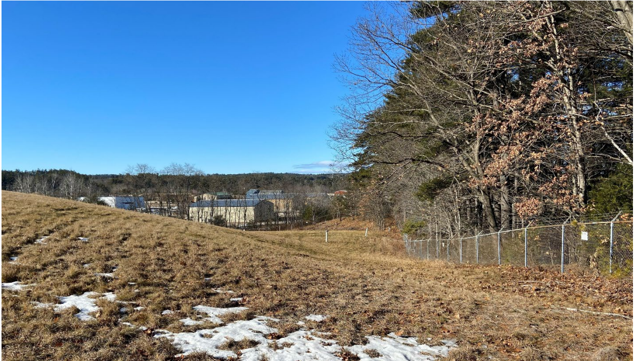
Photo 3: Stable and established slopes in inactive, capped area of landfill. The photograph was taken from near the top of the filled area and looking north.
